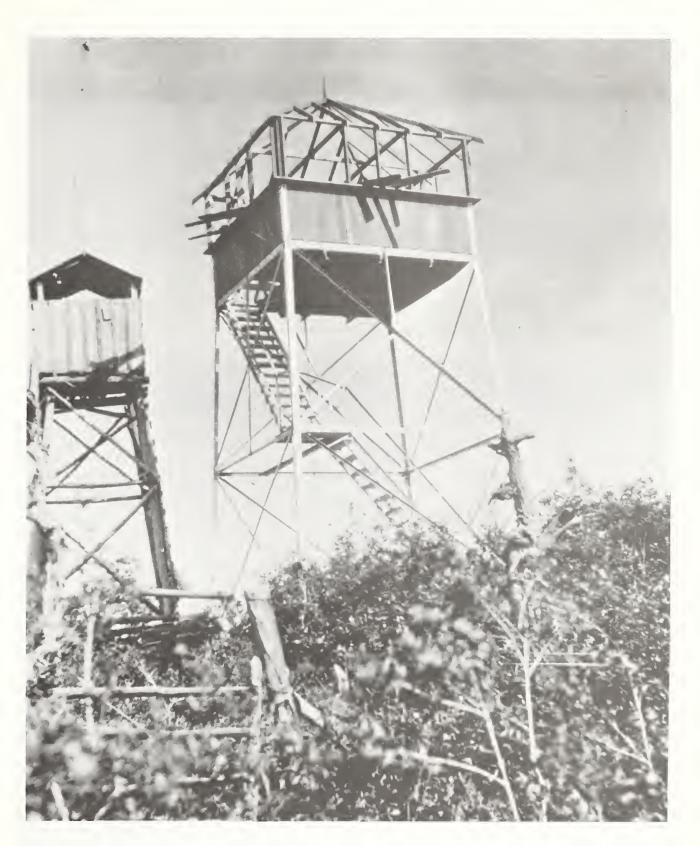
Figure 41. Rose Peak lookout tower, an Aermotor MC-24, under construction with the older wooden tower in the background. The site is on the Gila National Forest, New Mexico. Photo by I. B. Lash in 1928 (U. S. Forest Service photo 233862).
